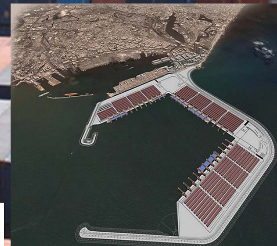
Colombo South port development (under construction)
